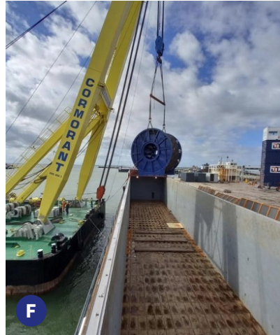
D Support vessel operating on site E Onshore cable crossings F Cable transportation from the Netherlands with a coaster
