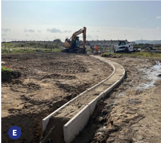
D Support vessel operating on site E Onshore cable crossings F Cable transportation from the Netherlands with a coaster
