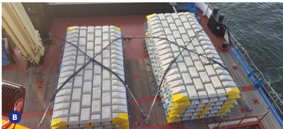
A Universal joint ready for over boarding B Mattresses ready for installation on cable crossing C Cable offloading at port of demobilisation D Over boarding Omega joint over boarding
